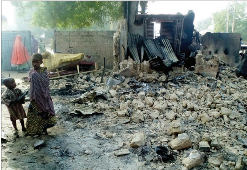
Children stand near the rubble of a house destroyed in deadly Boko Haram attacks in northeastern Nigeria in 2016.
