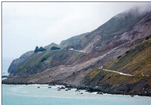
The roadway was severed by a massive landslide north of Ragged Point in Big Sur, California, May 25.
