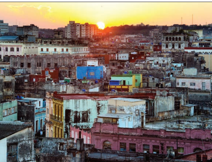
Havana's once-beautiful buildings are in a state of advanced decay.
