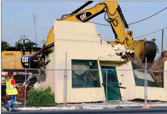
Fresno's Hollywood Bar makes way for HSR, July 14, 2014.
