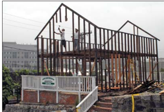
Disassembling the Kelo house (2007)
