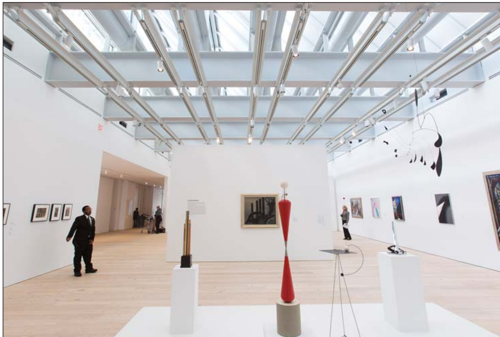
Eighth-floor gallery: exposed roof beams and slanted skylights
