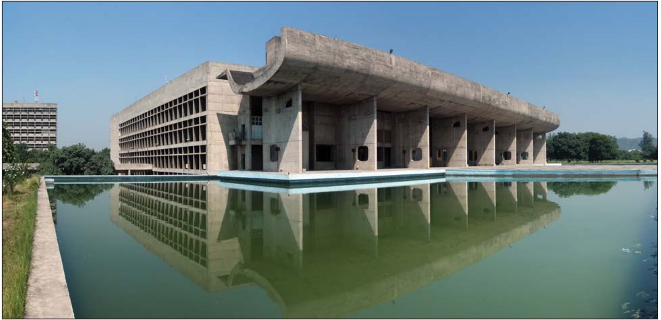
Le Corbusier's Palace of Assembly, Chandigarh
