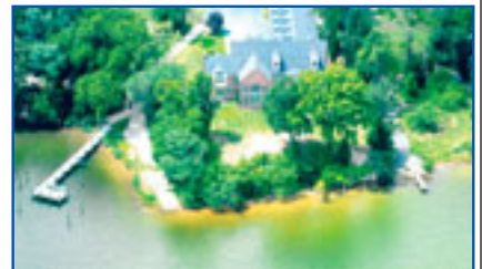
Custom Home All brick, including 4 bedroom and baths, 2-story, great room, foyer, first floor bedroom with bath. Over 5,000 square feet. Like new, 2 acres, 5 car garage, private pier with a ramp on point of land. Short sale.
