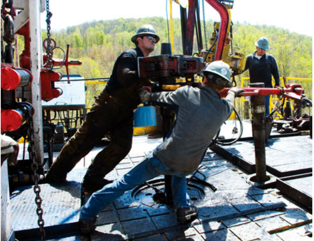
A Chesapeake Energy natural gas well near Burlington, Pennsylvania, April 23, 2010
