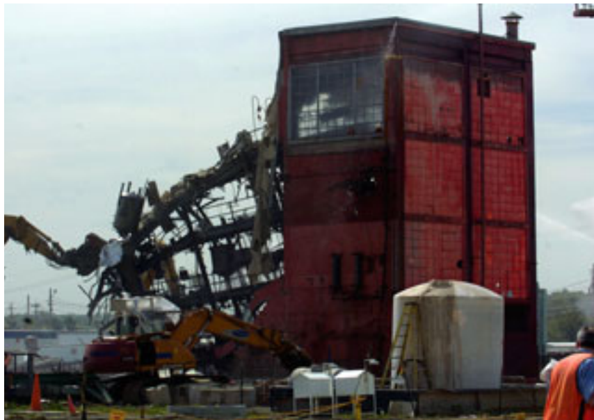
Demolition of a uranium production facility at Fernald, near Cincinnati, in 2004
