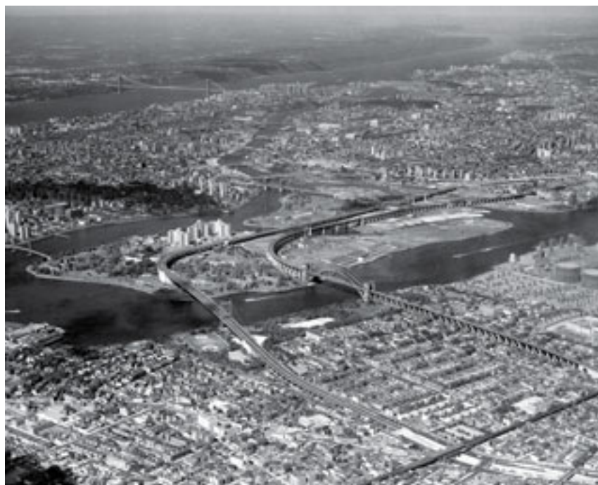
The Triborough Bridge, 1963
