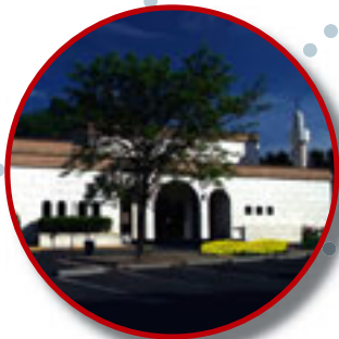
THE DAR AL HIJRAH ISLAMIC CENTER IN FALLS CHURCH
