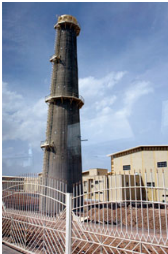
The Natanz nuclear enrichment facility south of Tehran
