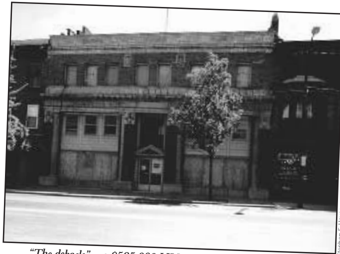
"The debacle"—a $585,000 HUD renovation in Albion, N.Y.
