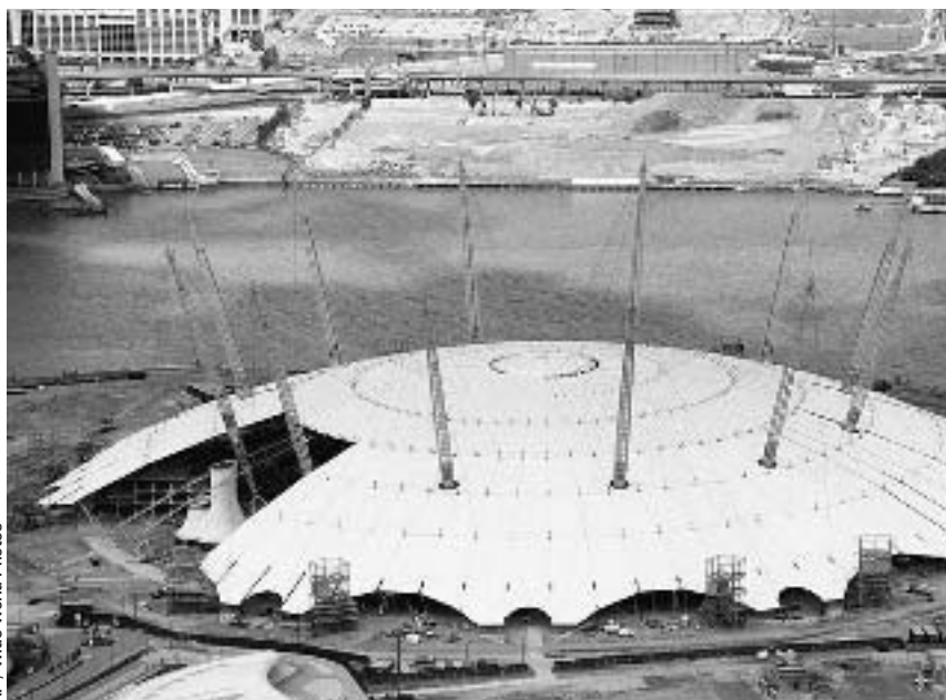
Construction of the Millennium Dome in London.
